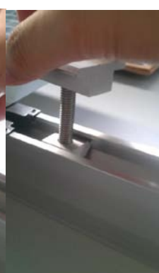
install inter clamp
