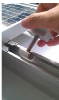
install inter clamp
